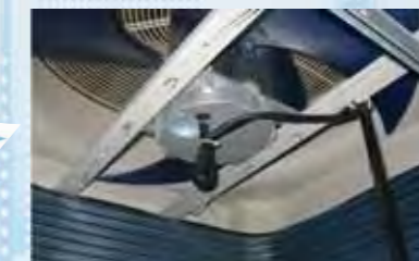
Every 20 seconds, compare the system pressure and the best pressure to adjust DC fan motor speed timely.
