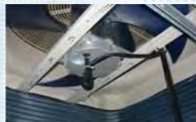
Every 20 seconds, compare the system pressure and the best pressure to adjust DC fan motor speed timely.
